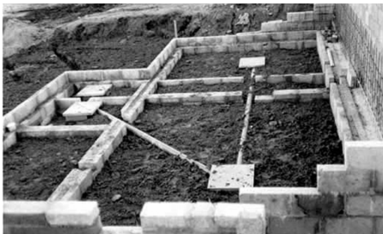
Sumps prior to pouring concrete floor slab
